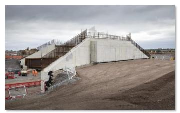
*Figure 3 : The image above shows the abutments and wing walls for the East West Rail Overbridge.*
