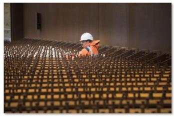
*Figure 3: The image above shows preparations taking place for the concrete element of the composite deck for the East West Rail Overbridge, November 2022.*
