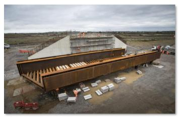
*Figure 3: The image above shows the assembled steel deck in preparation of the superlift, carried out in early December 2022.*
